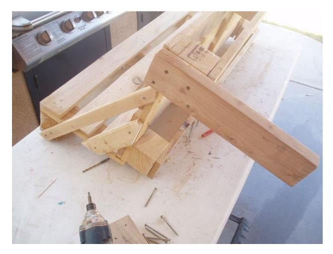
I wanted my bench to be  $16^{\prime\prime}$  from the ground. I measured and cut each 2x4 at  $16^{\prime\prime}$  then attached them to the sides both on the front and back for support. I used 4,  $3^{\prime\prime}$  screws to anchor the legs to the bench.
